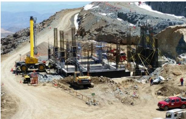
With the placement of steel reinforcement in support columns and beams, the summit building has begun to emerge from the foundation.
