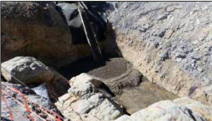
**Left: Concrete being poured for the platforms to be used as the foundation support of the building columns and floors for the LSST support building on Cerro Pachón. The effort used 1,210 cubic meters of concrete to level the site below the column footings.**
